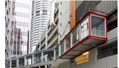
Equinix SE3 IBX data center exterior
