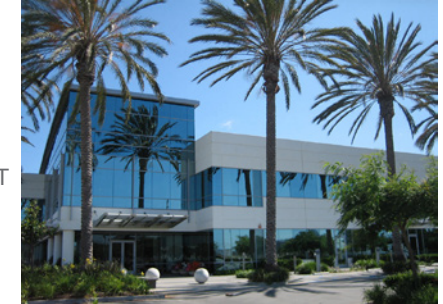
Equinix LA4 IBX exterior
