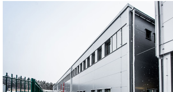
Equinix SK2 IBX data center exterior
